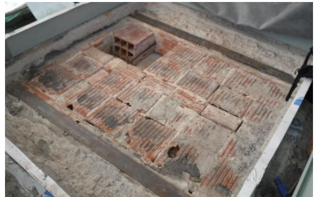
Hollow Terracotta Tile Floor Assembly
