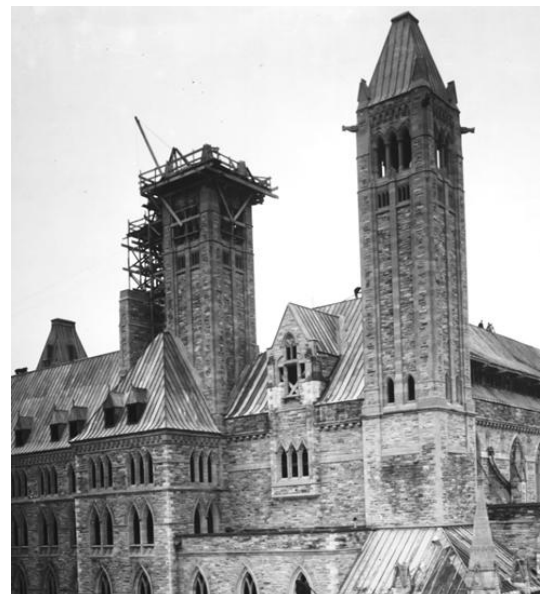
Centre Block's West Water and Ventilation Towers under construction (1918)
